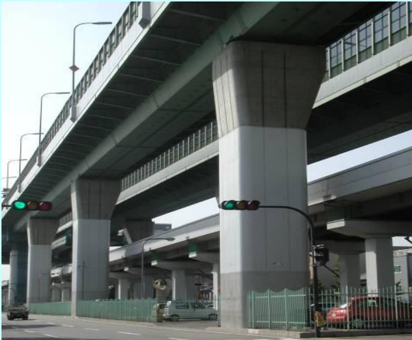
Pier of Hanshin Expressway
