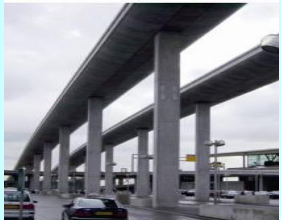
Charles de Gaulle Airport Pier on access road
